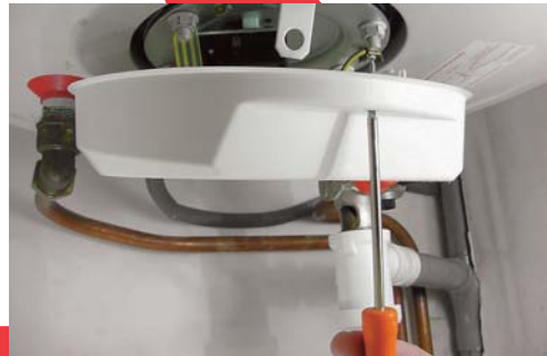
2 - Retirez le capot de protection.
